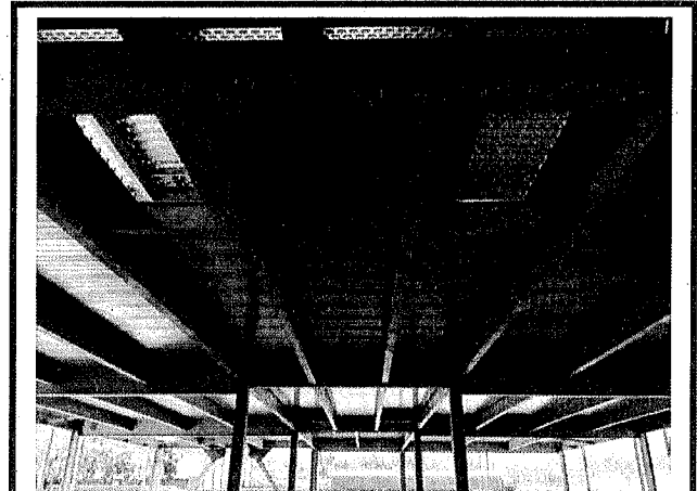
Metal Deck on Bldg B
