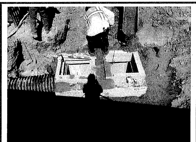
Bio-Clean Vault Placement
